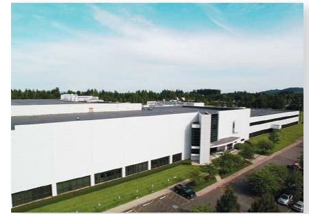
Gresham, Oregon: With more than 200,000 square feet of clean room space, this is Microchip's most technically advanced manufacturing facility. Today, the facility produces 8 inch wafers on 0.5 micron process technology with the capability to support process technologies down to 0.13 micron.
